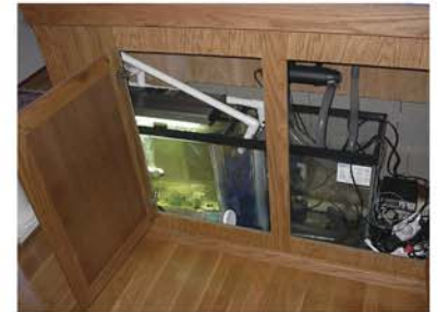
Cabinet Based Filtration
